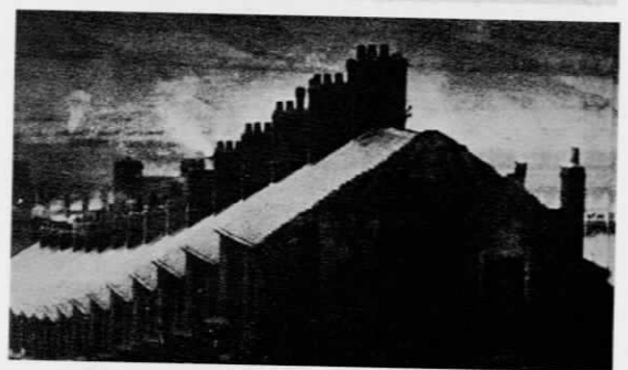
16 Le Corbusier, La Ville Contemporaine, project, 1922 17 Mies van der Rohe, Patio houses, floor plan, 1938 18 Row houses from Victorian times, Newcastle upon Tyne, England
